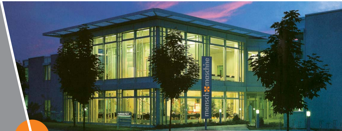
The M+M headquarters in Wessling near Munich
